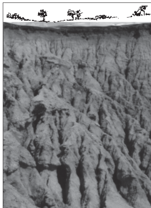
Soil erosion in New Caledonia
