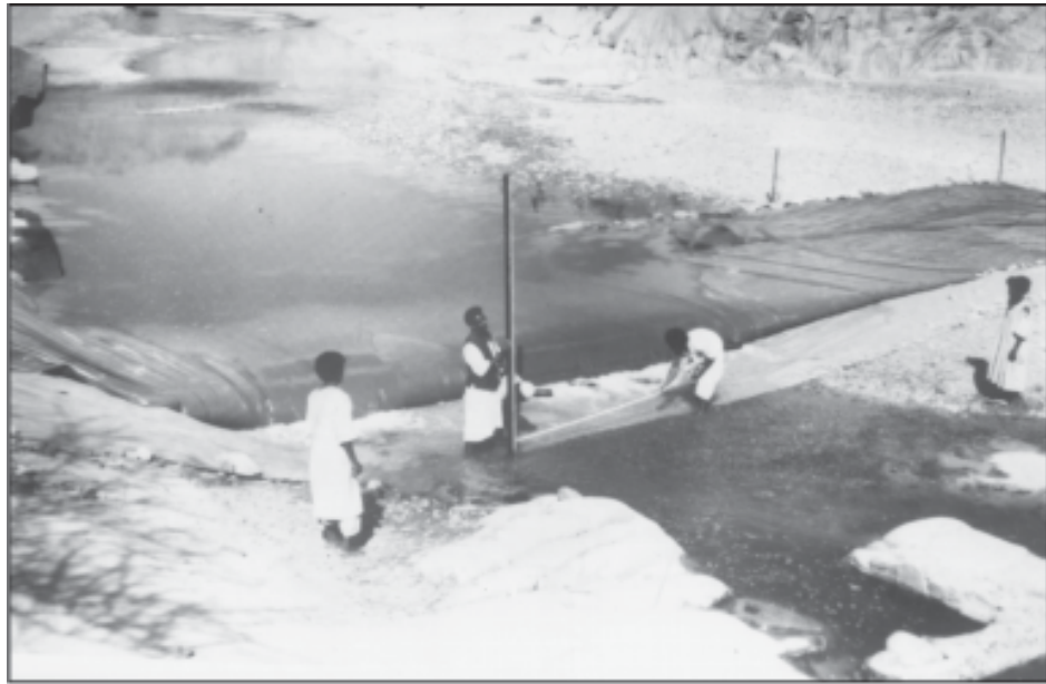
A new type of inflatable rubber dam used to help irrigation in very dry areas
